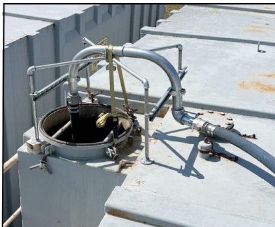
Anti-Siphon Manhole Light Cage Mounted on Frac Tank
