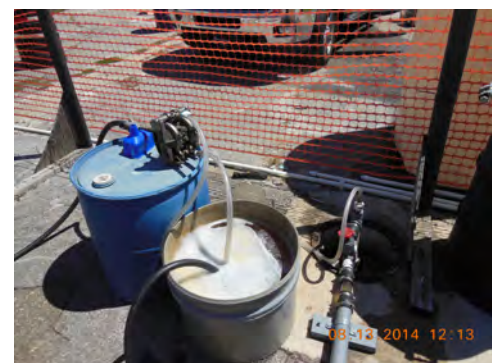
HC-2000 Injection into Extraction Wells
