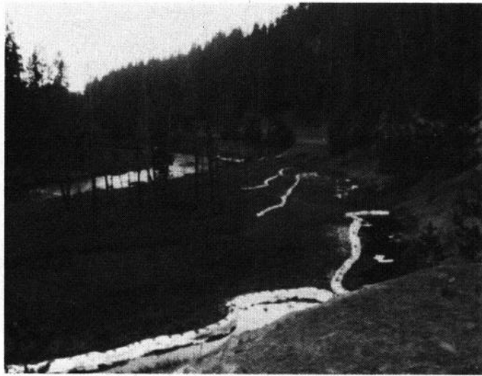
Polypropylene sorbent barriers contain gasoline residues and direct plume migration toward the toe of the roadbed.
