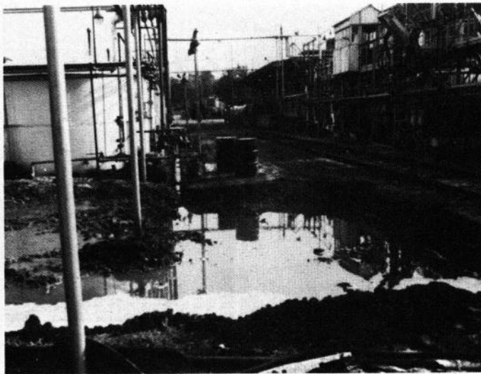
Tank farm spill of monononylphenol, 810 alcohol, and solvents contaminated groundwater and leached into a nearby stream.
