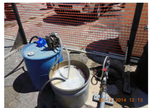
HC-2000 Injection into Extraction Wells
