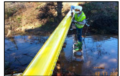
Split Casing Containment with Leak Detection on Fuel Line Over Stream
