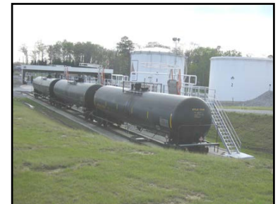
Ethanol Unloading Rack with Secondary Containment
