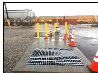
Pre-Cast Oil Containment Weir Box, Hydrocarbon Sensor & Automated Sluice Gate
