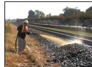
HC2 Fuel Remediation on 1800 ft of Rail w/o Track Time
