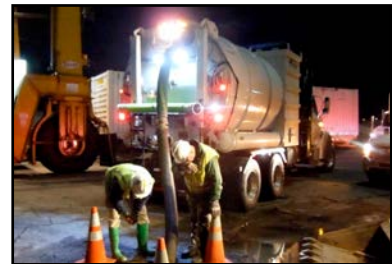
Vacuum Fuel Extraction from Leaking Line in Railyard
