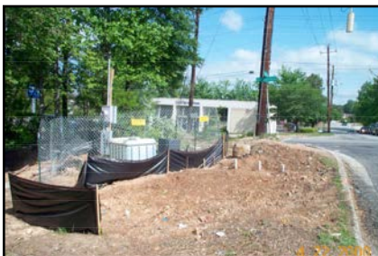
HC2 Diesel Spill Remediation around 100 yr old Fragile Water Main
