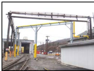
Construction of Fuel Pipe Bridge with Secondary Containment
