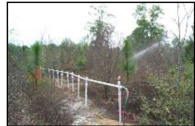
HC2 Gasoline Wetland BioFence Remediation System
