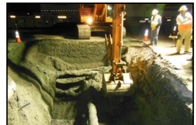
Leaking Fuel Cleanup & Line Repair
