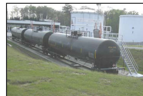
Ethanol Unloading Rack with Secondary Containment
