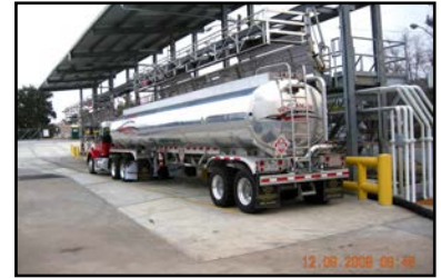
Loading Rack with Secondary Containment & Gantry Access
