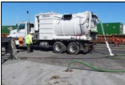
Total Fluids Fuel Extraction at Railyard Pipeline Break
