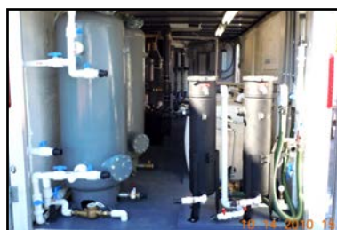
Remtech Mobile Vacuum Extraction System at Diesel LUST Site
