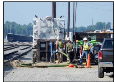
VacuJET TM Removes Heavy Sludge From 300 ft 24" Sewer Sections
