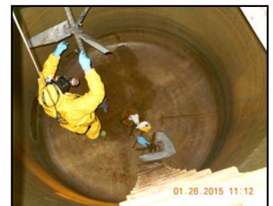
Mixer Blade Repair in Reactor
