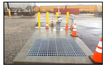
Stormwater Oil Containment Weir Box with Automated Sluice Gate & Hydrocarbon Sensor
