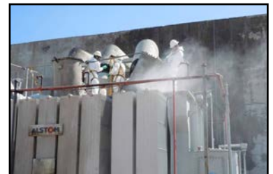
Steam Cleaning 250 MW Transformer after Fire
