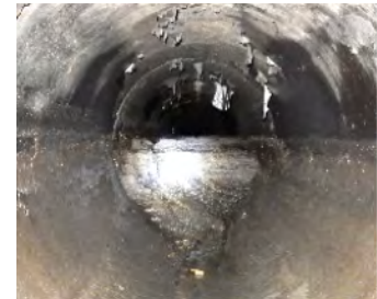
Solids in Sewer Prior to Cleaning
