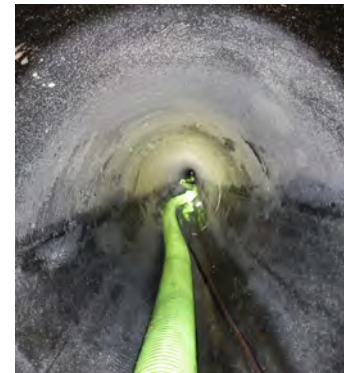
VacuJet™ Cleaning Process Evacuates Solids from 300 ft Sewer Sections
