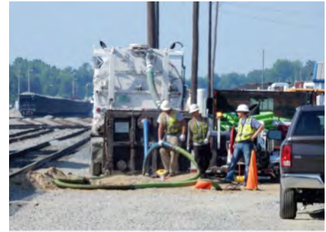
VacuJet At Vacuum & Jetter Hose Feed at Lead Manhole
