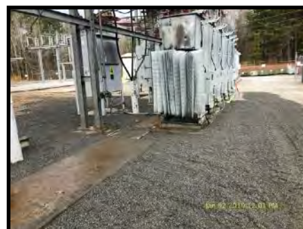
Completed Substation Pad with Clean Gravel
