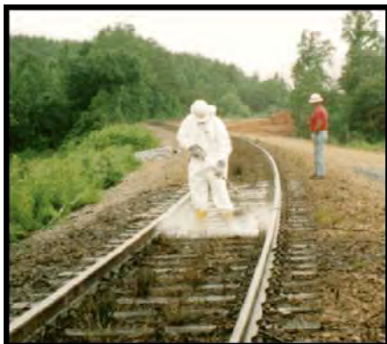
HC-2000 Track Bed Application
