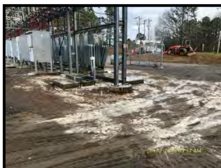
Grounding Grid Soils and Metal and Concreted Pads Treated with HC2
