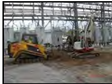
Excavate Saturated Soil Above Grounding Grid
