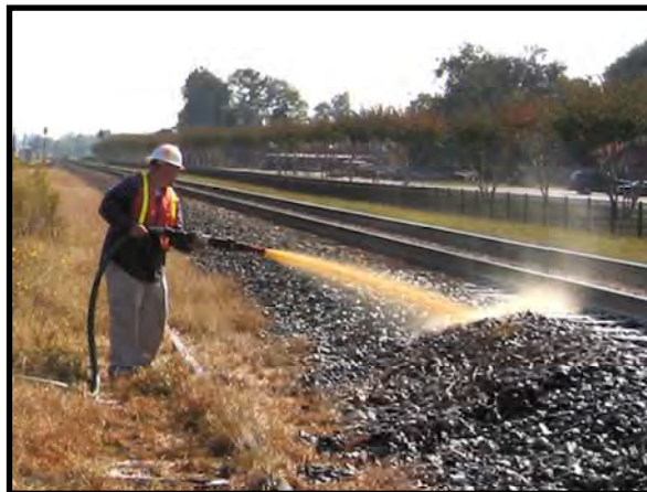
Application of HC-2000 to Track Siding
