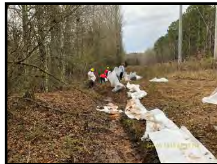
Removal of Free Product with Poly Sorbent
