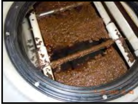
Heavy Iron Bacteria in OWS From Wells Closest to Bay 1
