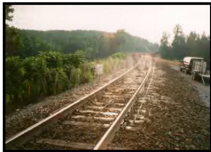
Solar Powered Water Mist Application
