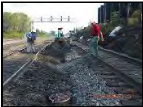
Leachate Collection System Installed Between Tracks
