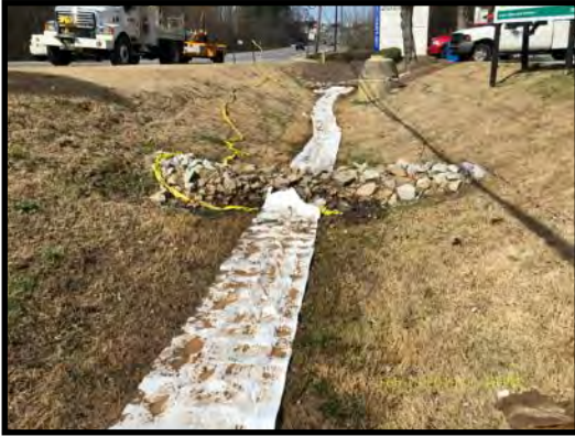
Polypropylene Sorbent Removes Bulk Mineral Oil
