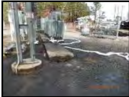
Remove Free Product and Saturated Gravel
