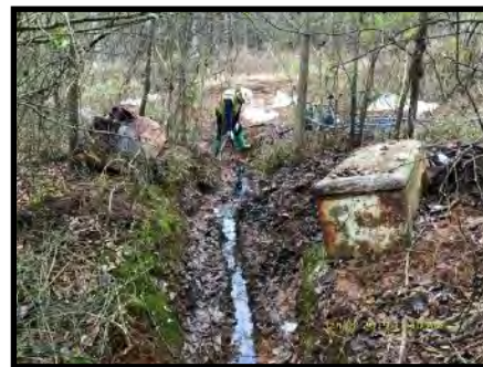
Recovery of Oil from Storm Drain and Desorbed Oil from Ditch Soil
