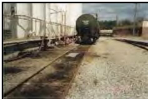
30 Years of Lube Oil Accumulation on Ballast Reduced by Over 60% After Four (4) Months of HC-2000 Treatment
