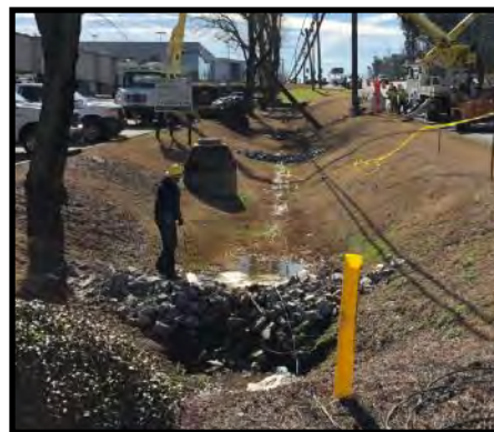
3 Transformers Landed in Drainage Ditch Releasing 40 Gal of Transformer Oil
