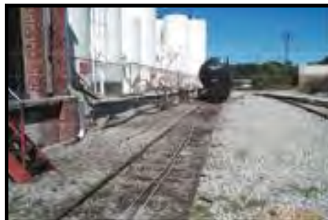
30 Years of Lube Oil Accumulation on Ballast Reduced by Over 60% After Four (4) Months of HC-2000 Treatment
