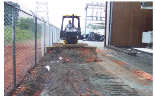
Excavation of Grossly Contaminated Soils above Grounding Grid
