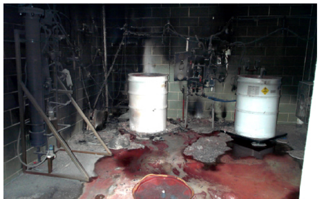
Explosion in Chlorine Dioxide Generation Room
