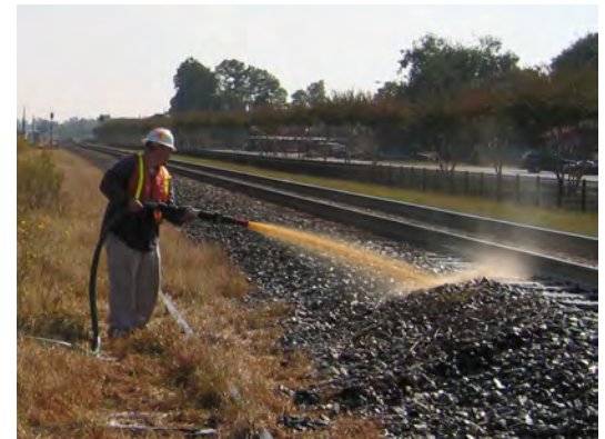
HC-2000 applied to track cross sections with fire nozzle from access road
