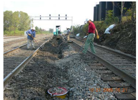
Installation of Leachate Collection System between Mainline Tracks
