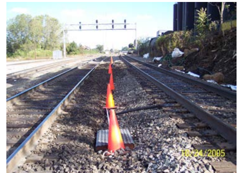
Leachate Collection & Straw/Sorbent Ditch Containment Systems
