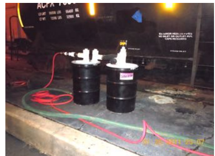
Remtech Carbon Off-Gas Scrubbers
