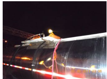
Pneumatic Transfer of TDI to Stainless Tankers
