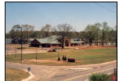
Arsenic Contaminated Foundry Site Remediated During Construction
