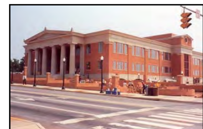
Gasoline in Fractured Rock under $16M Building Remediated During Construction
