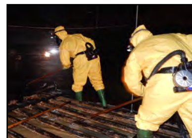
Tank & Heating Coil Cleaning
