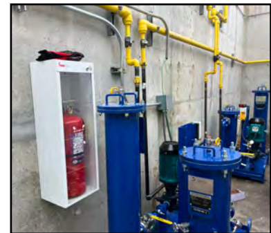
Fuel Conditioning System Installation
