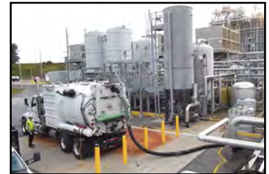
Contaminated Gravel Removal
