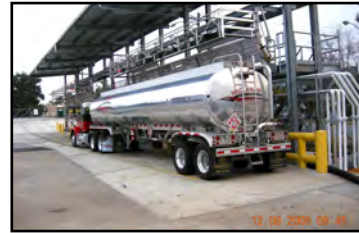
Loading Rack with Secondary Containment & Gantry Access
