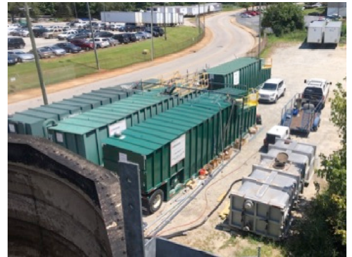
Emergency 60,000 gal Aerated Equalization Basin with Micro Bubble Diffusion
