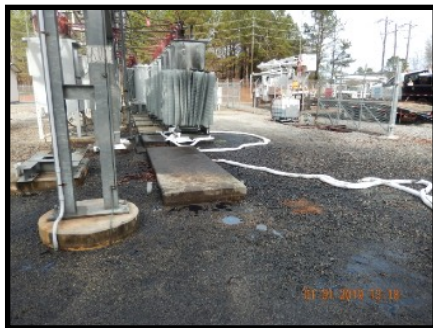
Remove Free Product and Saturated Gravel
