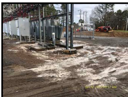
Grounding Grid Soils and Metal and Concreted Pads Treated with HC2
