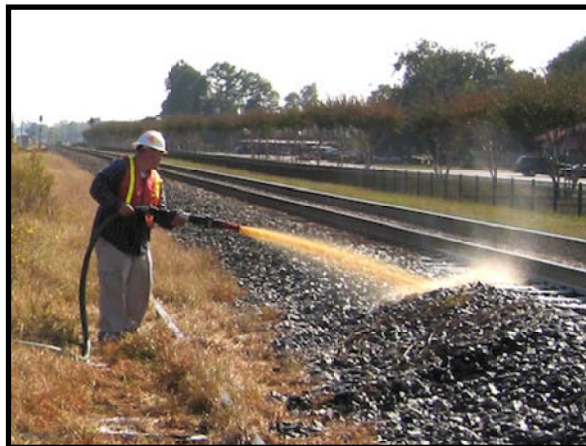
Application of HC-2000 to Track Siding
