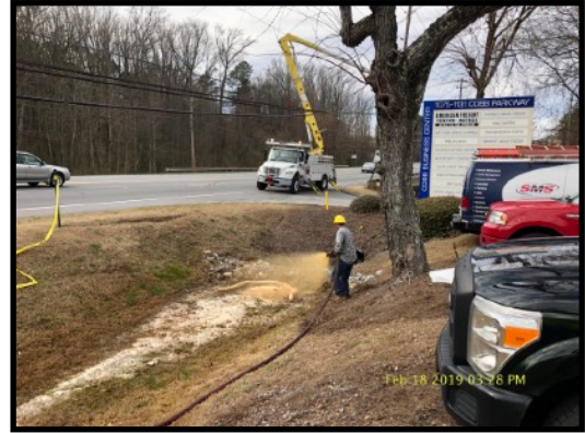
HC-2000 Sprayed on Grass to Desorb Additional Oil and Accelerate Degradation
