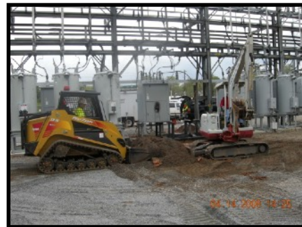
Excavate Saturated Soil Above Grounding Grid
