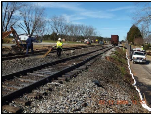
HC-2000 Application to Diesel Impacted Ballast
