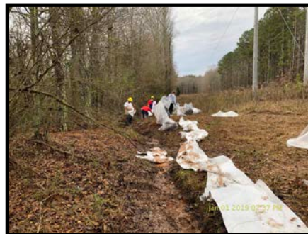
Removal of Free Product with Poly Sorbent
