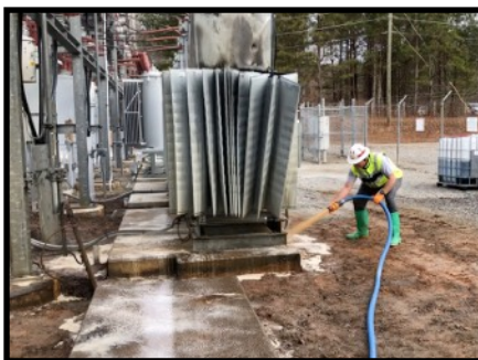
Clean Metal Superstructure and Treat Grounding Grid Soil with HC-2000
