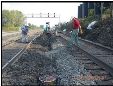
Leachate Collection System Installed Between Tracks
