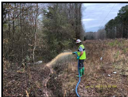
HC2 Application to Desorb Soil from Drainage Ditch
