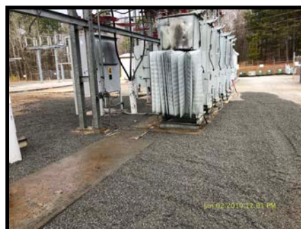
Completed Substation Pad with Clean Gravel
