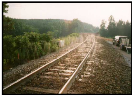
Solar Powered Water Mist Application
