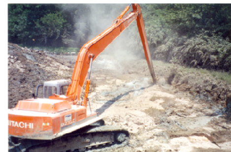
Chemical Fixation of Wastes Drives off VOCs
