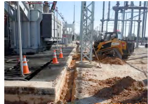
Excavation of Contaminated Soils
