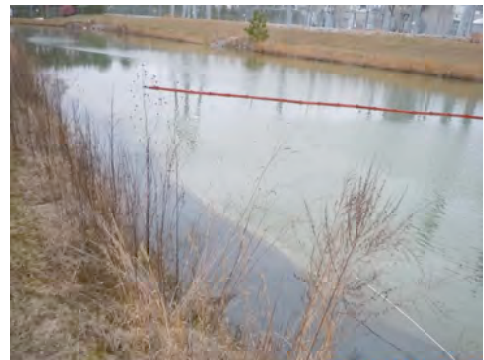
Removing Free Product from Detention Basin
