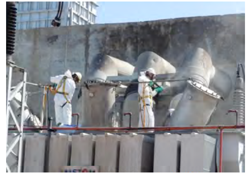
Steam Cleaning Transformer Shell
