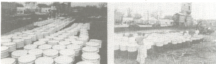
Figure 7. Contaminated residues packaged in 17H drums. 485 drums were loaded using front-end loaders and transported by covered trucks for ultimate disposition.
