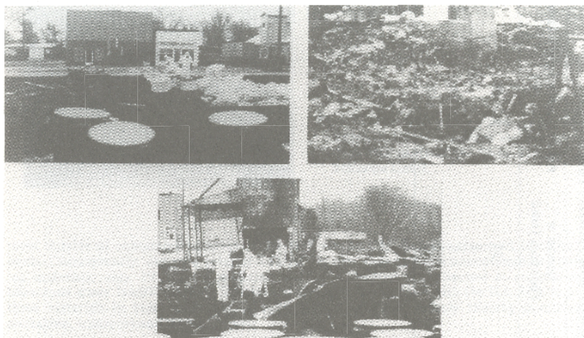
Figure 6. REACT personnel packaging Dyanap soil residues, Treflan residues and white Atrazine residues contaminated soil. Packaging operations of Atrazine and Treflan residues using polyethylene bags placed in 17H epoxy lined drums.
