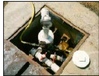
HC-2000/BioSparge Injection Well at Gasoline GUST Trust Fund Reimbursed Site
