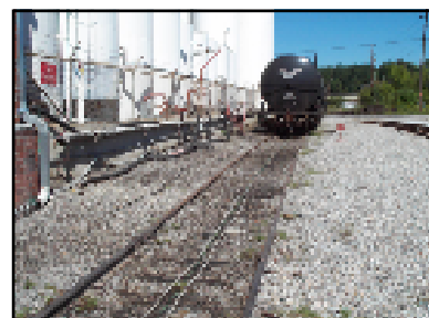
Ballast Staining & Oil Concentrations Reduced by 70%+ after 4 months of HC2 Treatment
