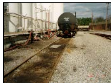
Motor Oil Contaminated Ballast Before HC2 Treatment
