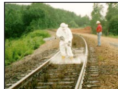
HC2 Degrades Diesel Fuel & Odors in Railroad Ballast w/o Track Time
