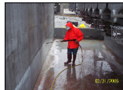
Transformer Oil Removed from Containment Structure at Power Plant
