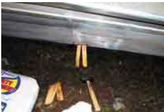
Wood Braces Hold Epoxy Putty Stopping Leak in 8,000 gallon Diesel Fuel Tanker
