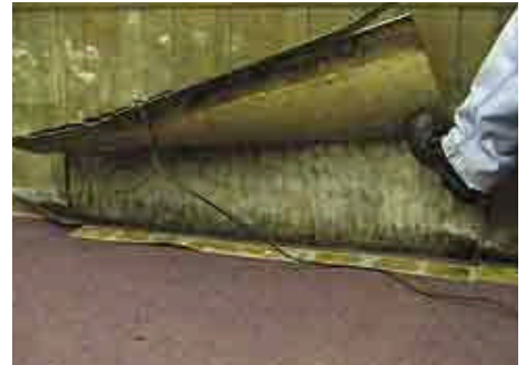
Mold Growth Behind R & D Facility Paneling
