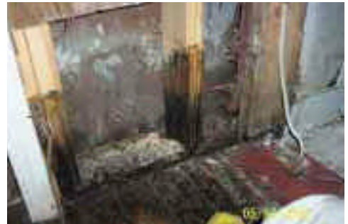
Mold Growth on Wood Studs
