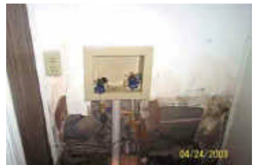
Mold in Wall Cavity from Water Line Break
