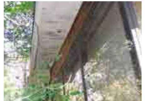
Mold Attacks Soffit from Roof Leak
