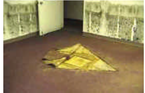
Extensive Wall and Flooring Mold Damage
