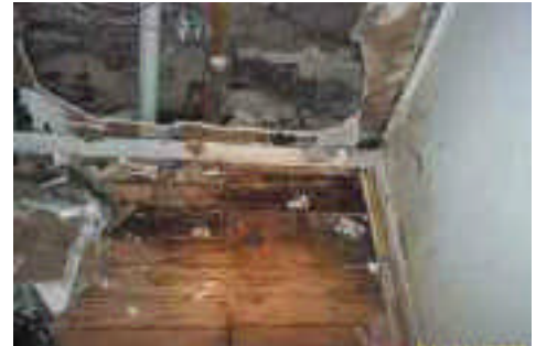
Mold Attacks Wood Subfloor
