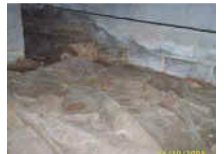
Block Wall Seepage Causes Mold
