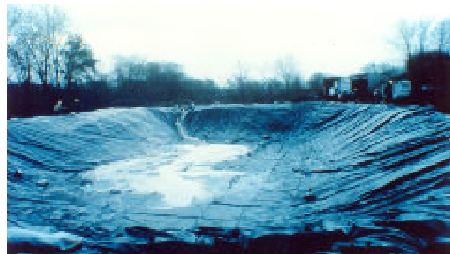
300,000 gal. Treatment Lagoon for Stream Fire Leachates
